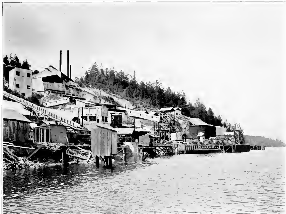
Cement-works, Portland Cement and Construction Co., under Construction at Bamerton, Sannick Arm.
